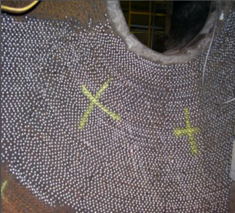
➤ T5 studs on neck wall
